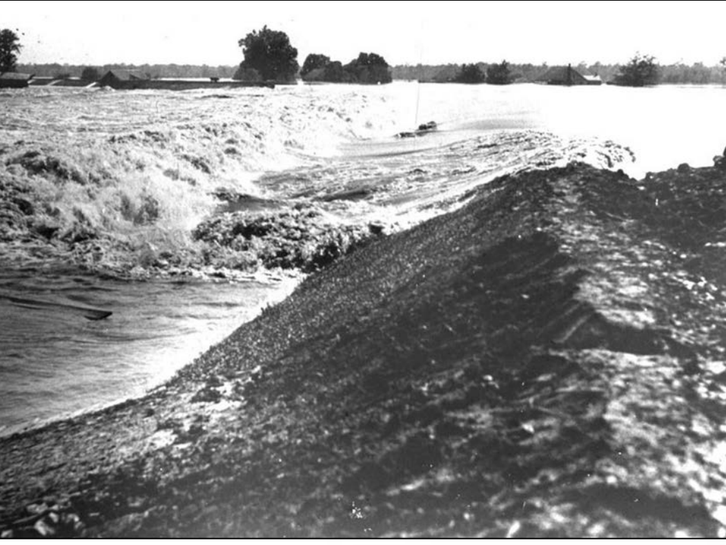
< Levee breach along the Mississippi River near Bordelonville, Louisiana, 1927. Source: University of Chicago Library.
